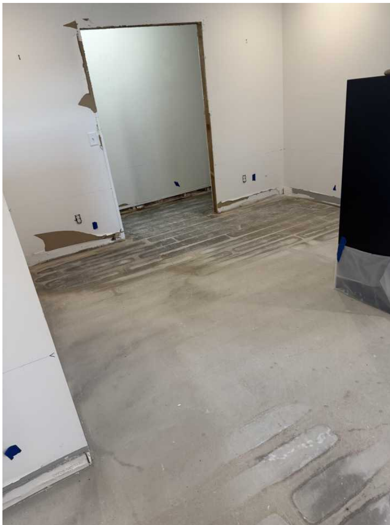
23 23-Bedroom demo progress Date Taken: 2/10/2026
